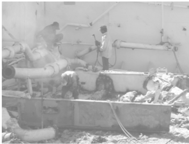
Fig. 12 Workers take out asbestos and glass wool from engine room of scrapped ship without having any protective tools (Photo: Author,2004)
